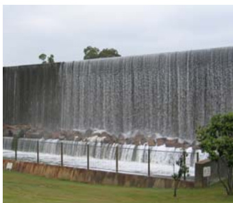
Foam in the attenuation weir
