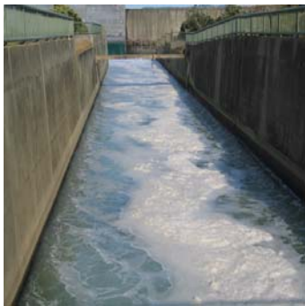
Foam in the Eraring Power Station outlet canal
