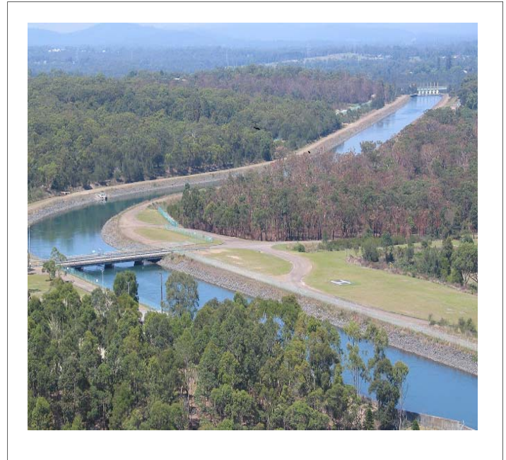
Eraring Power Station Inlet Canal
